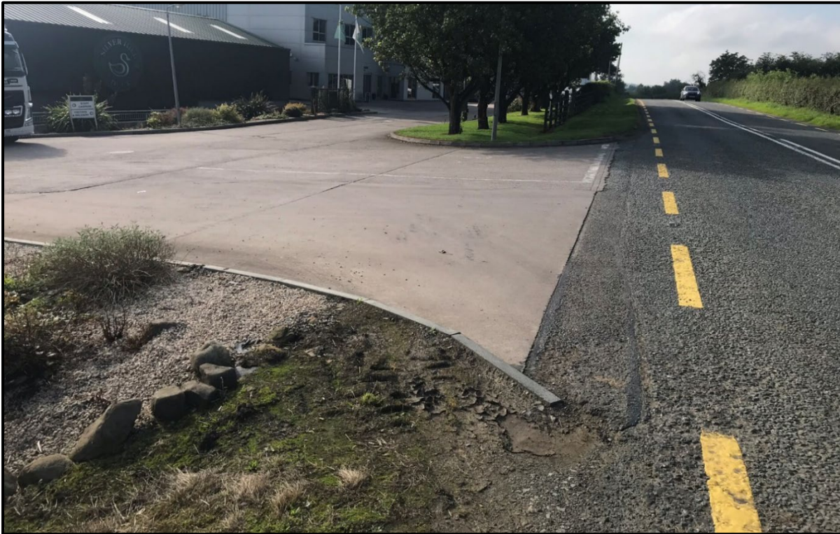
Figure 3.2 – View of site access junction along N2 travelling south towards Emyvale
