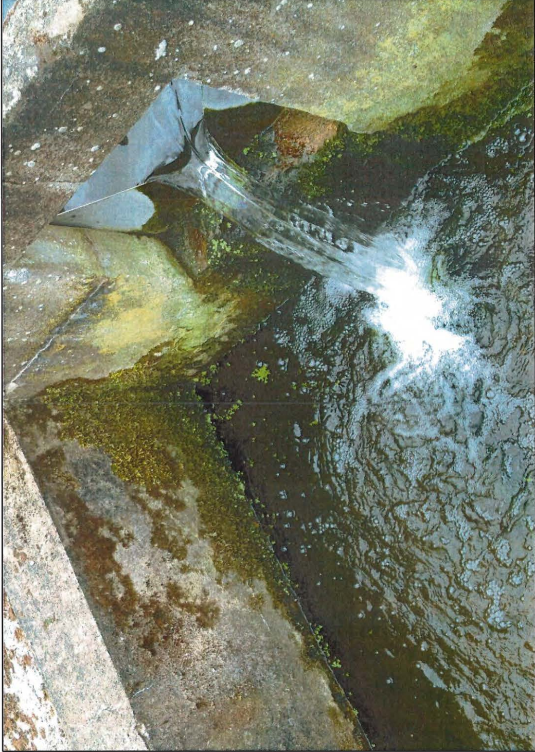
Photo of current final discharge point SW1 (V-notch)
